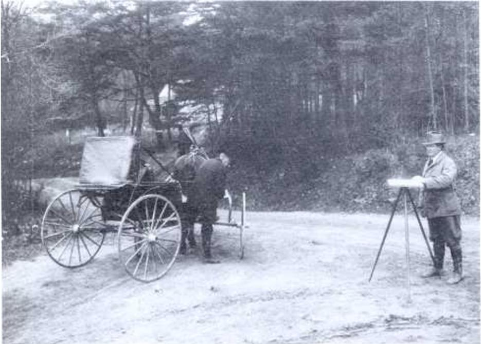
Specimen field operations in soil surveys in the United States in 1914. One man is reading the odometer next to the right front wheel of the buggy while the other is prepared to sight back along the road segment just traversed and then mark the new location on the field sheet as soon as he gets the distance covered. The photograph also illustrates the common plane table plus acceptable field clothes of the period. USDA photograph.
