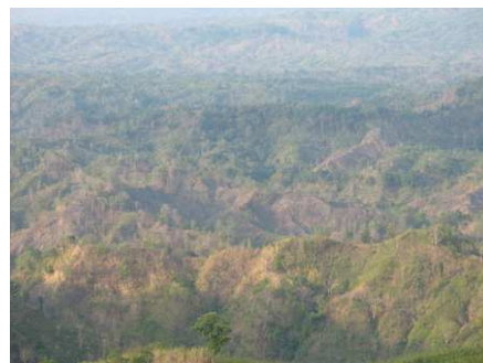
A view of site 'A'
