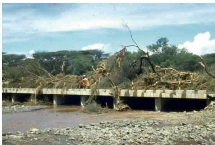
Figure 5 Debris and sediment fills reservoirs Photo: WOCAT
